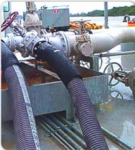
Hose in service; note the gradual bend achieved off of the horizontal connections
